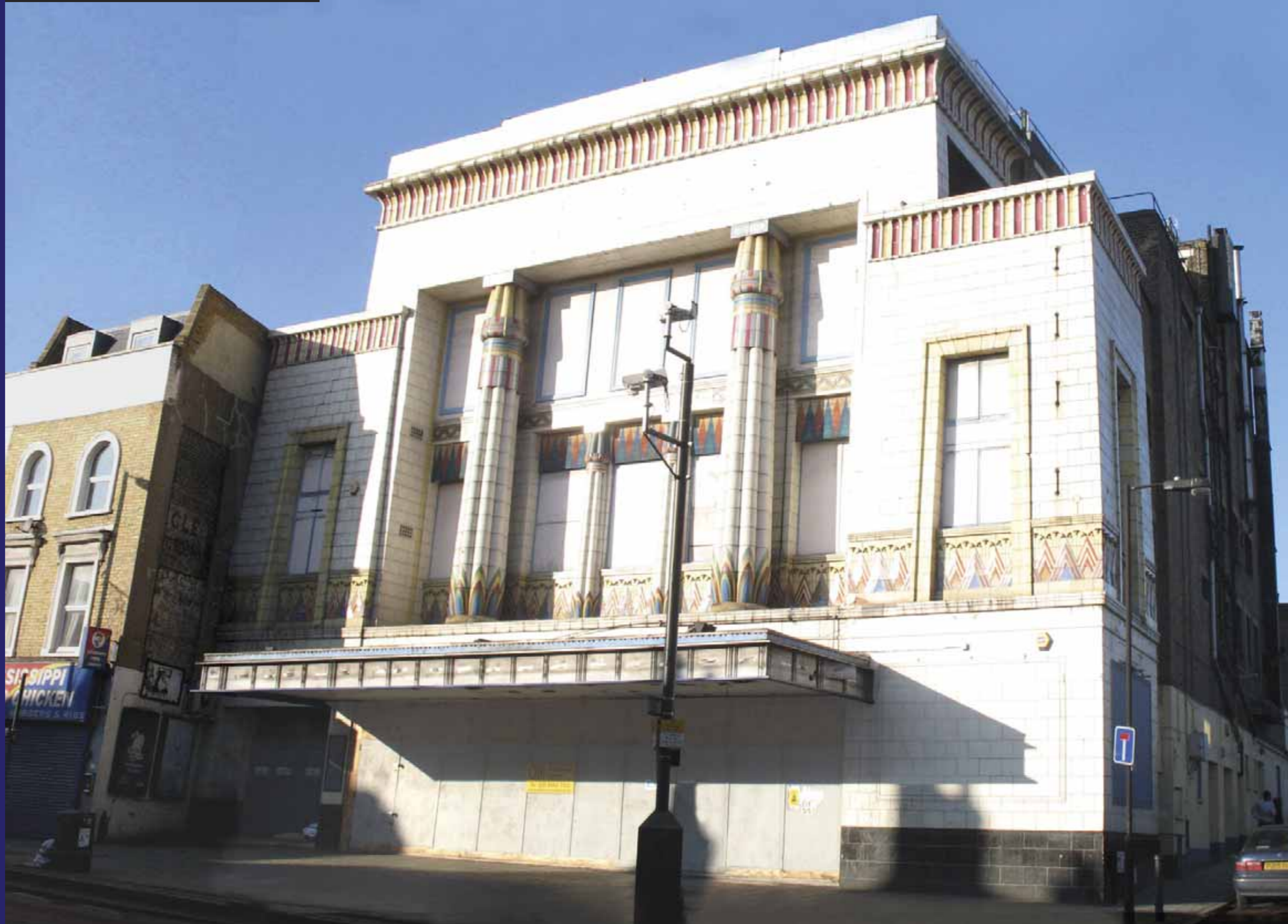
The existing building
